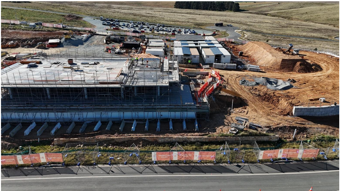
Image caption: Construction is progressing on Block B
